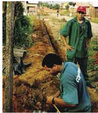
View of Condominial Water Branch
