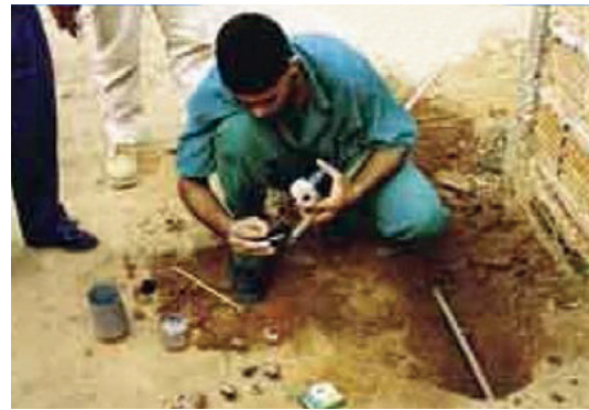
Installation of micro-meter in household connection, Parauapebas
