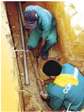
Installation of the Public Water Network
