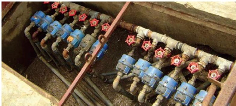
Meter chamber on Line 1
